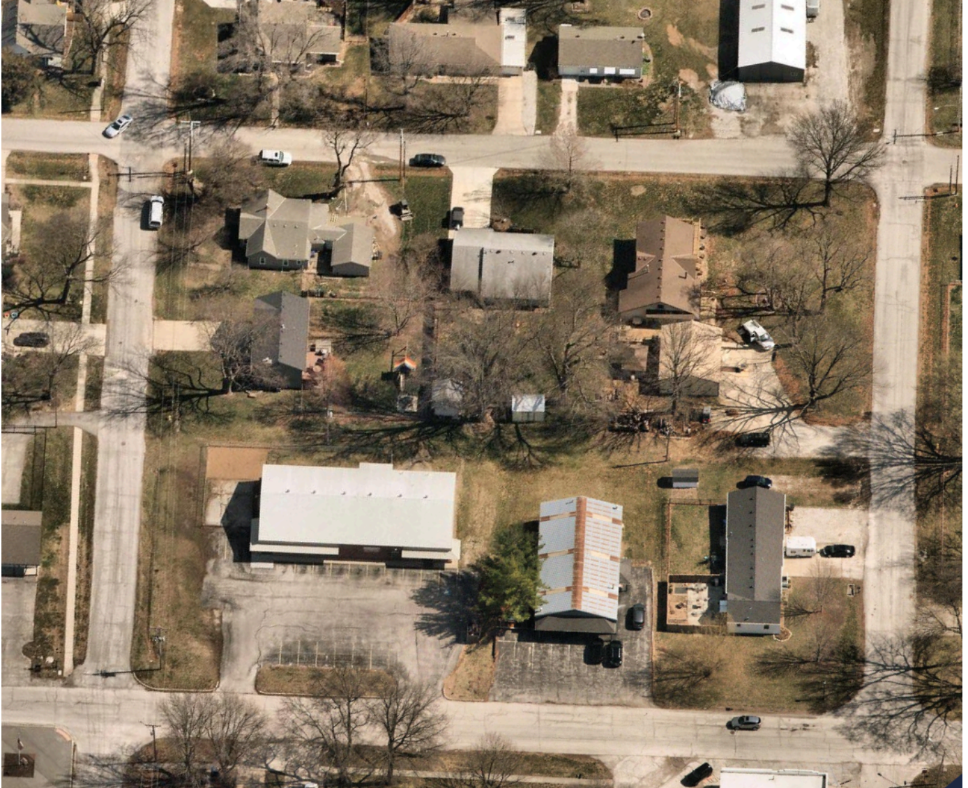
Aerial view looking east from Washington Street (Nearmap)
