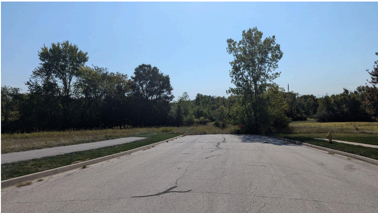
View looking south at the terminus of Elk Drive, proposed for future extension.
