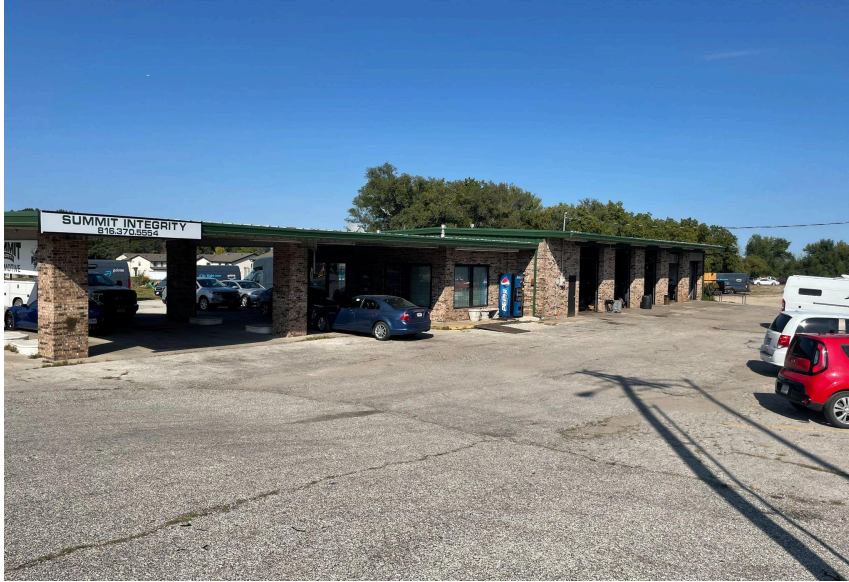
View looking northeast from southwest property corner.
