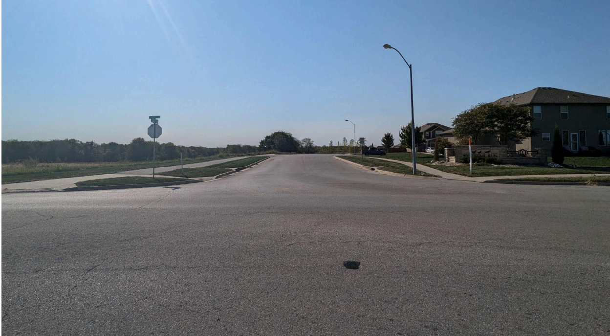
View looking south along Elk Drive entering into White Tail Run. Existing development on the right, proposed development area on the left.
