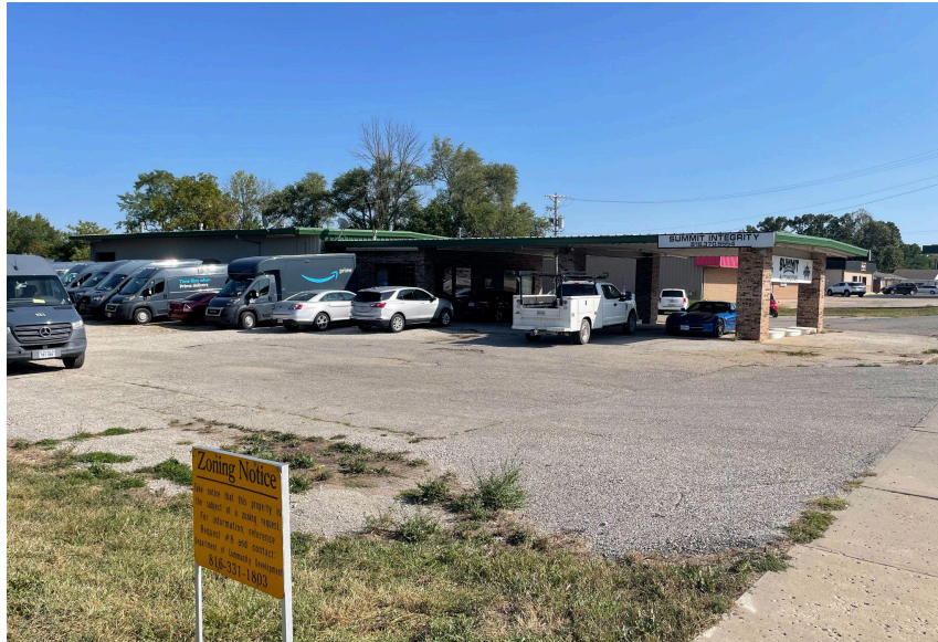
View looking southeast from northwest property corner.
