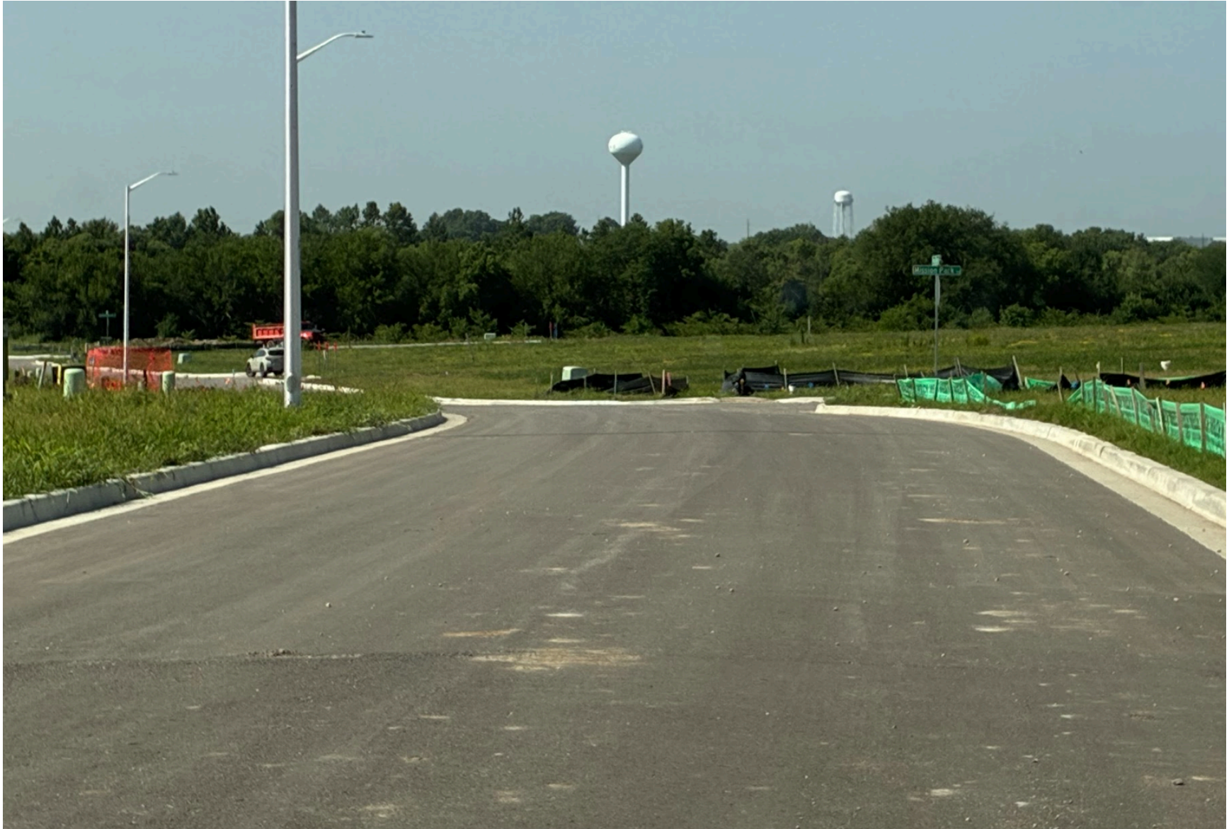
Looking South from Sendera Subdivision (Existing Tower on the Left)
