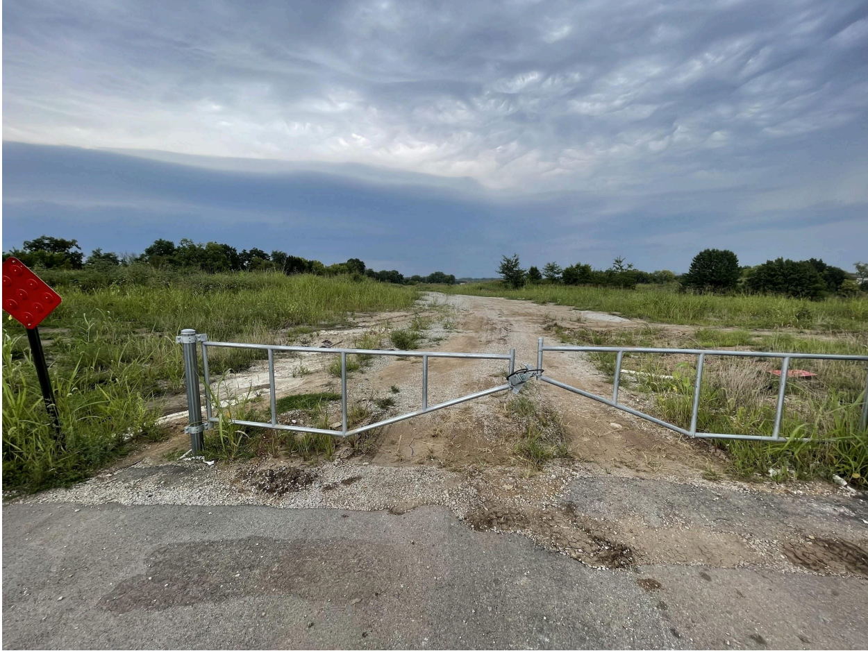
Looking North from Glenn Circle and Creekmoor Drive
