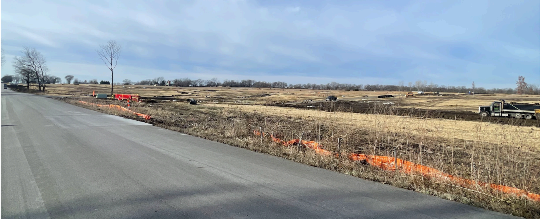
SE Corner Looking NW
