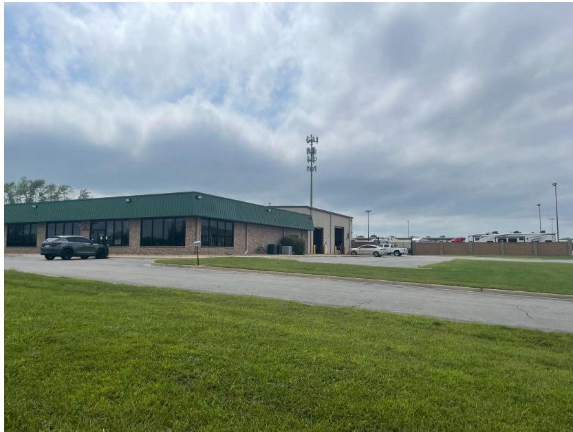
View looking southwest from S. Lincoln Rd. (NE Property Corner)
