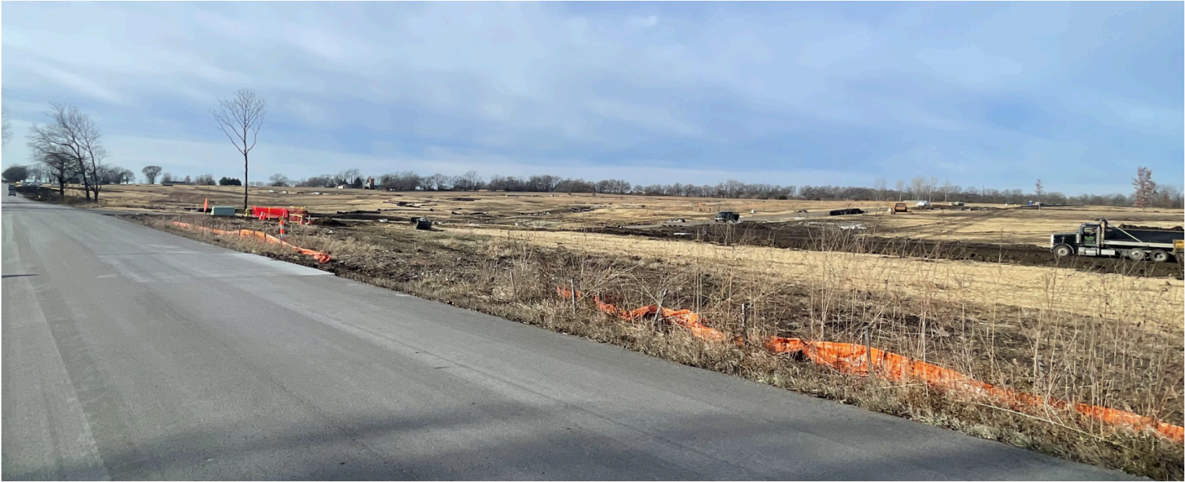
SE Corner Looking NW
