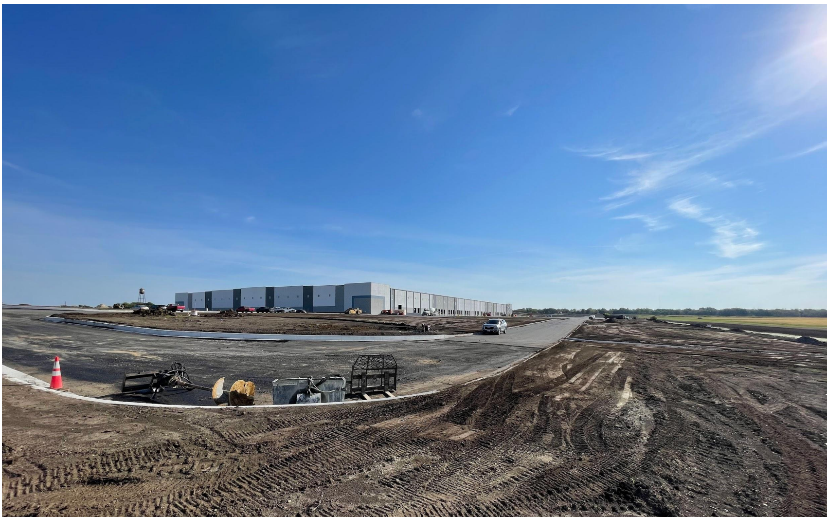
Near SW Corner of Lot 1 Looking NE
