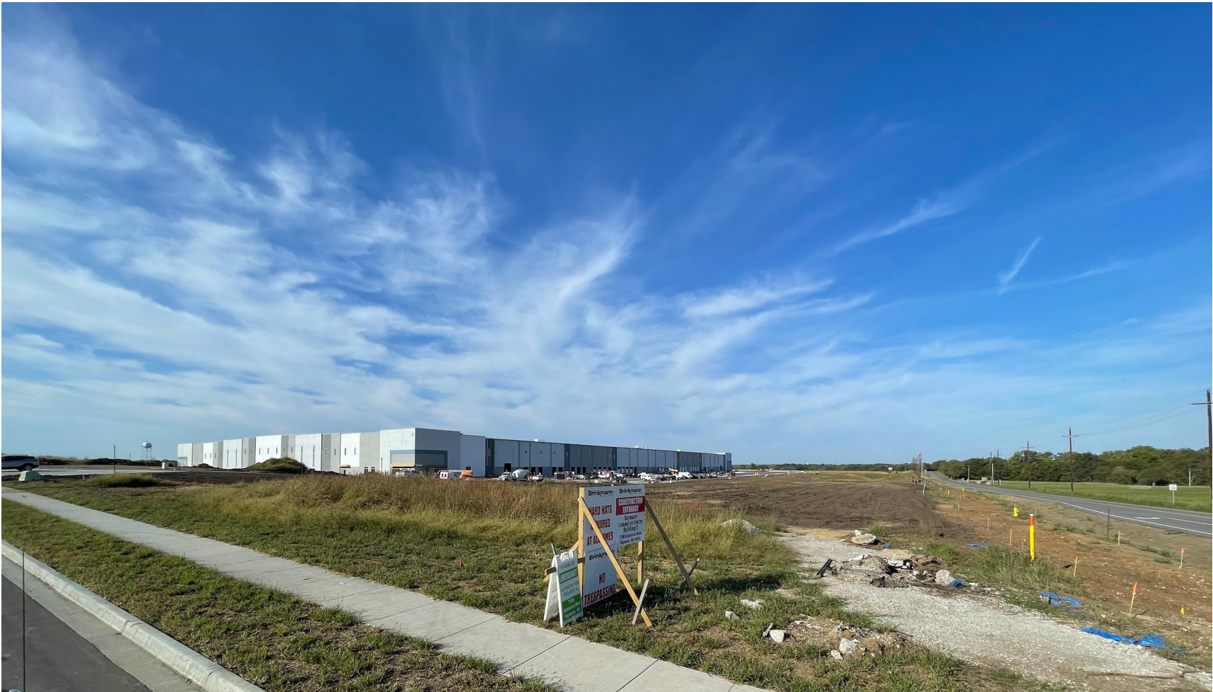
NE Corner of Lot 1 Looking SW
