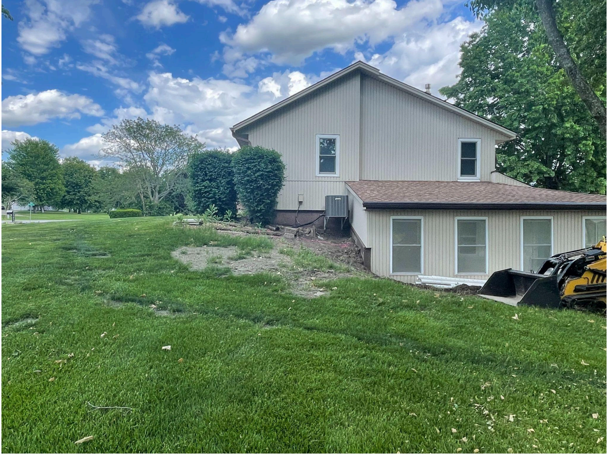
Looking east from west property line at west building facade (Sandpiper behind)
